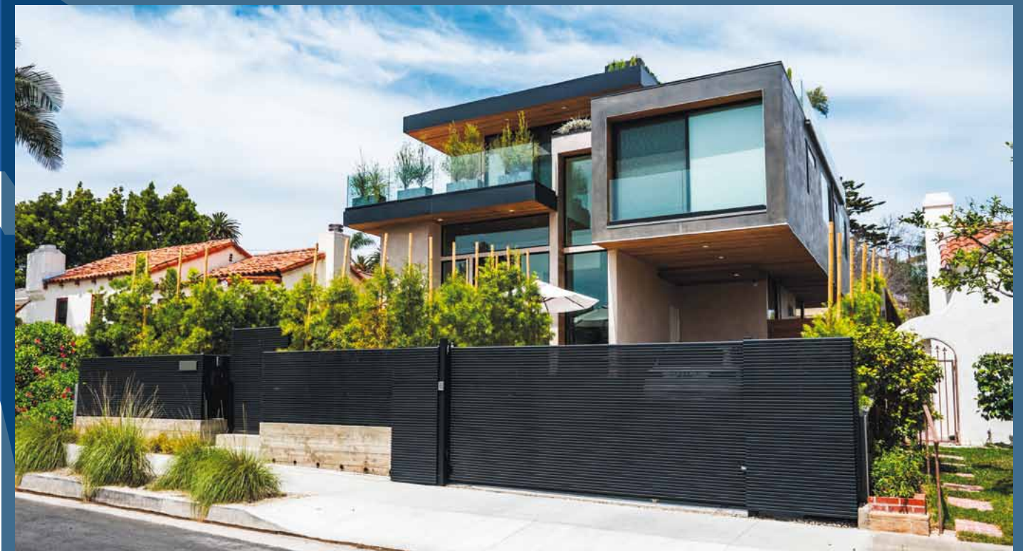
We created a security and privacy barrier to compliment this beautiful house in Mar Vista, California. May 2020
